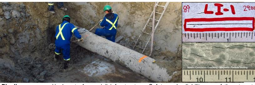
**Pipelines** are a critical part of our civil infrastructure. Safety and reliability are of the utmost importance. The potential for safety and environmental risks can be minimized through routine In-Line Inspections using Smart Tool Technologies. Problems identified using this technology need to be validated and assessed in the form or **Pipeline Integrity Assessment** digs.
